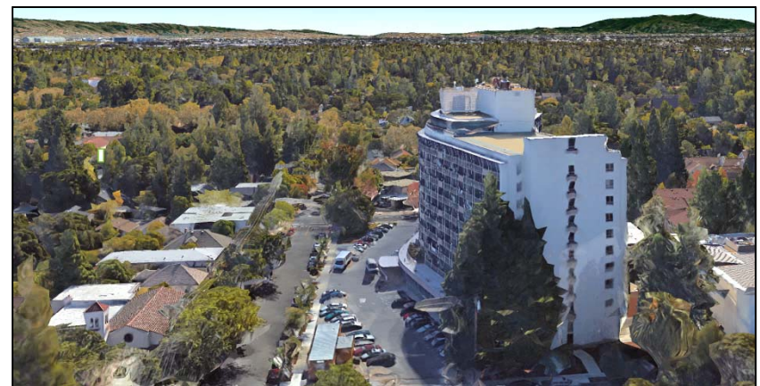
Channing House: Looking SW toward San Jose
