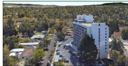
Channing House: Looking SW toward San Jose
