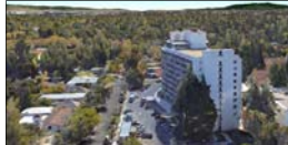
Channing House: Looking SW toward San Jose
