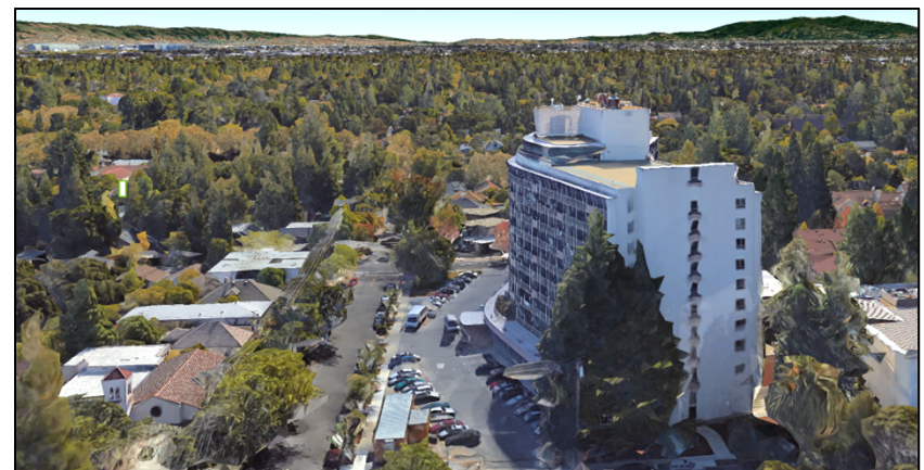
Channing House: Looking SW toward San Jose
